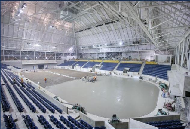
The picture seen here is a milestone for every hockey facility, the 'rink slab pour'. On a standard NHL® size rink surface, 9 miles of refrigeration piping is used and 220m<sup>3</sup> of concrete is required to pour the monolithic slab. It takes 6-8 hours to pour the concrete and another 10-14 hours finishing it so that one is left with the ideal flat slab.
