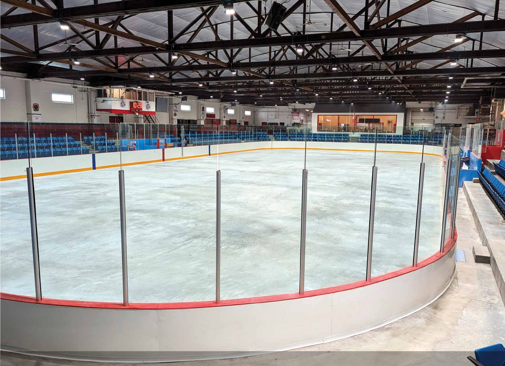
Ted Reeve Arena – Toronto, ON – Dasher Boards & Safety Netting
